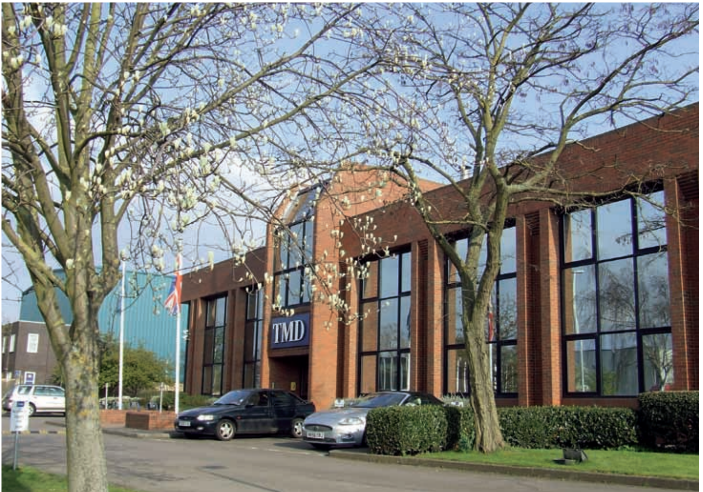
TMD's headquarters in Hayes, West London, where all departments work together as a team to achieve record results.
